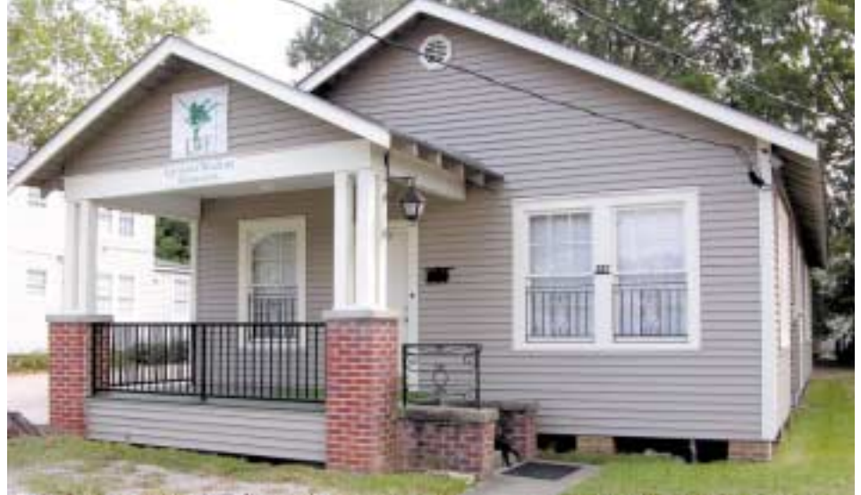
Louisiana Wildlife Federation office at 337 S. Acadian Thruway in Baton Rouge received a "facelift" this past summer with new siding and paint.
