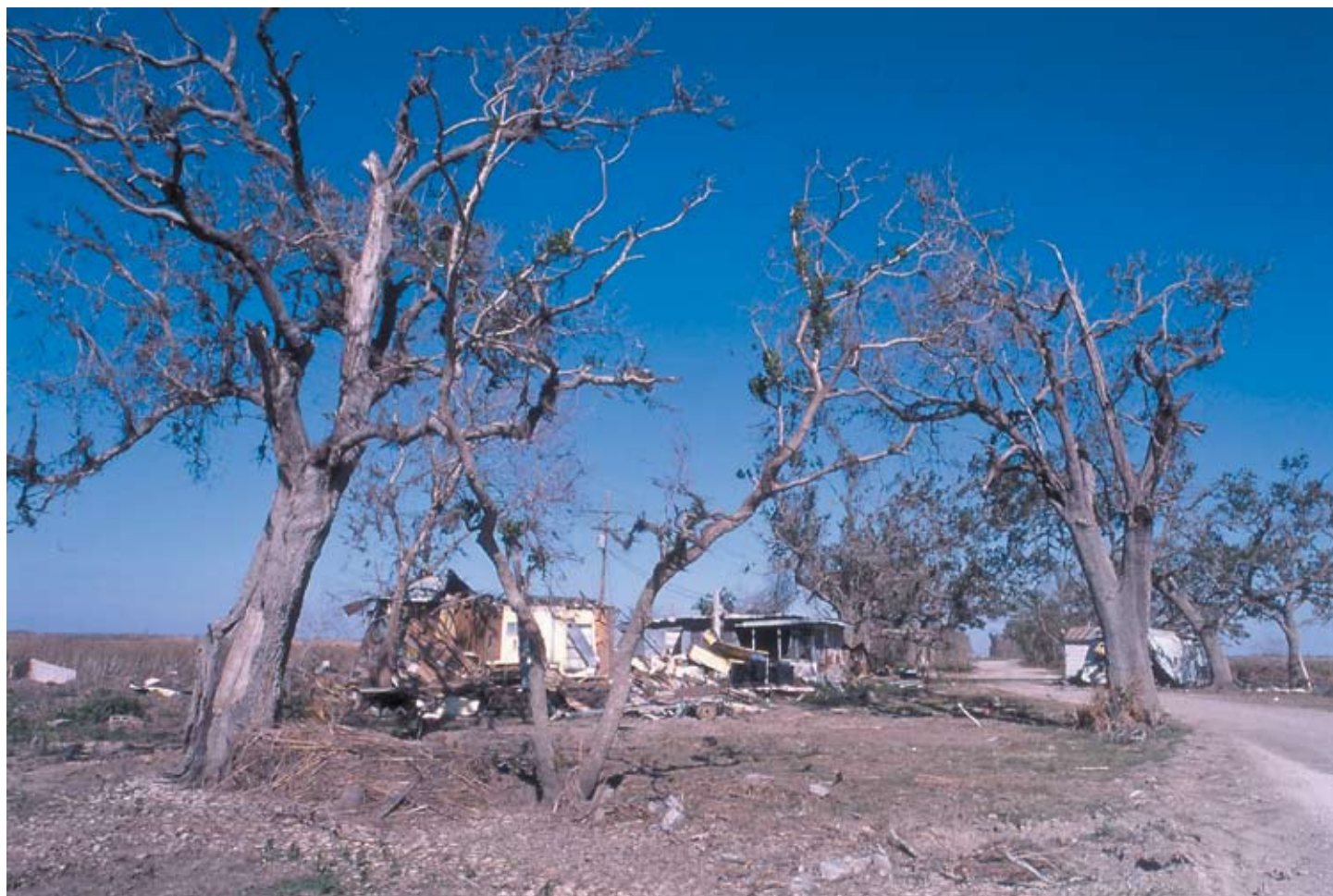
Hurricane Damage to oaks and dwellings on the chenier
