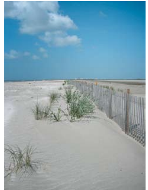
Grass planting and sand fencing between the Gulf and Bay Champagne to defend against storm surge over-wash.
